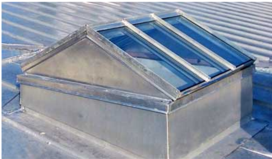
Figure 41. A gable ended double-glazed skylight installed at the restored US Marine Hospital in Louisville, Kentucky. Photo, New England Skylights
