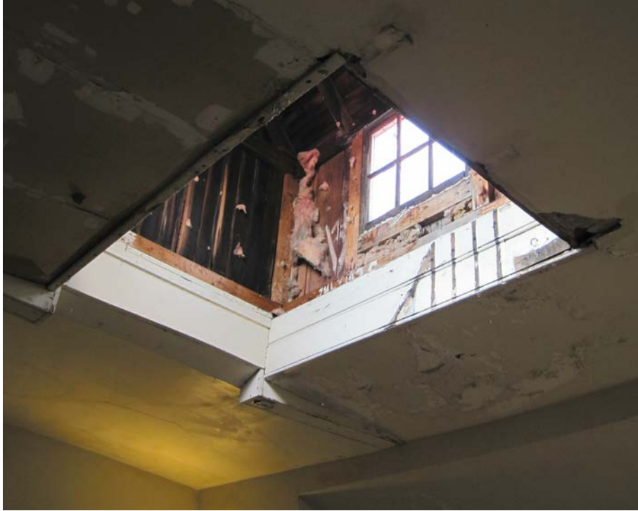
Figure 40. Interior of the present penthouse on a bright day. Note the need for supplemental lighting. Photo, Anthony Eardley, April 2010
